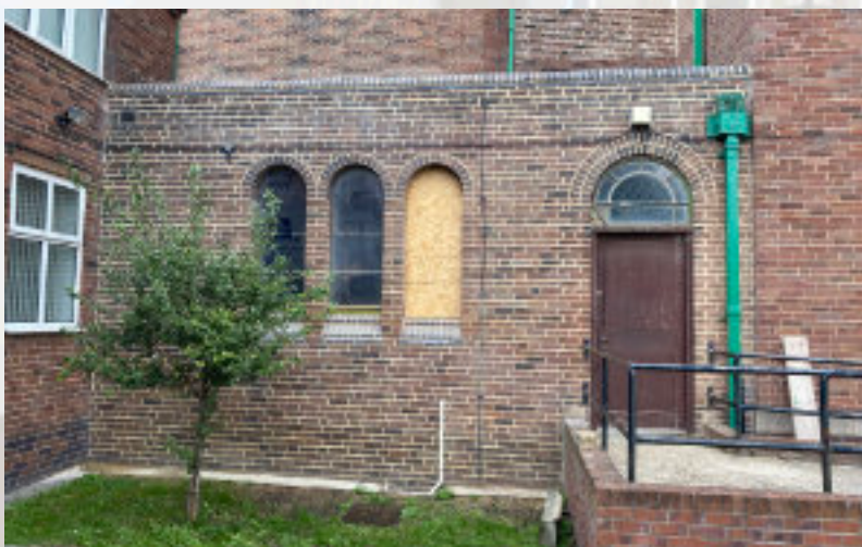
Outside the Sacristy: repointed brickworks and windows currently being restored
