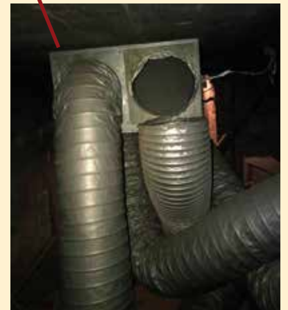
Disconnected ducts.
