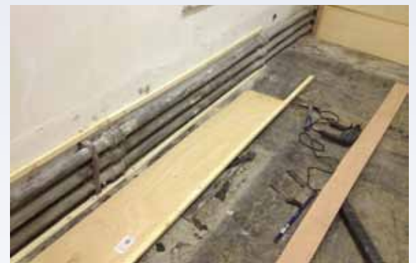
Covering the pipes from the antiquated heating system.
